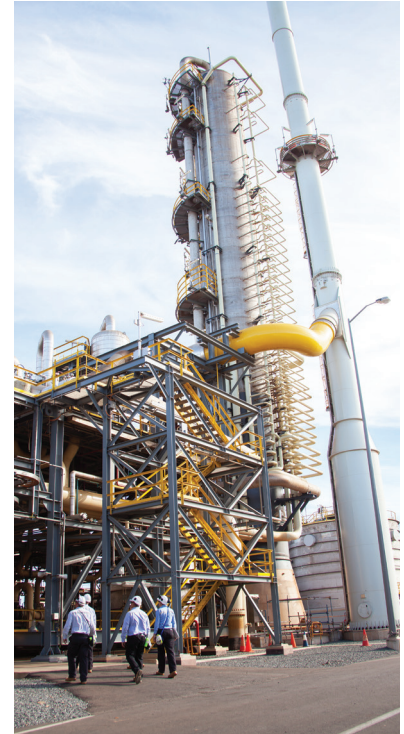
Yara Pilbara TAN Plant
