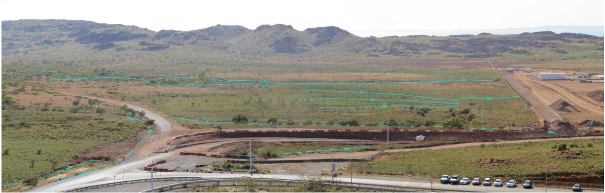
Figure 9-4 North West Creek diversion
