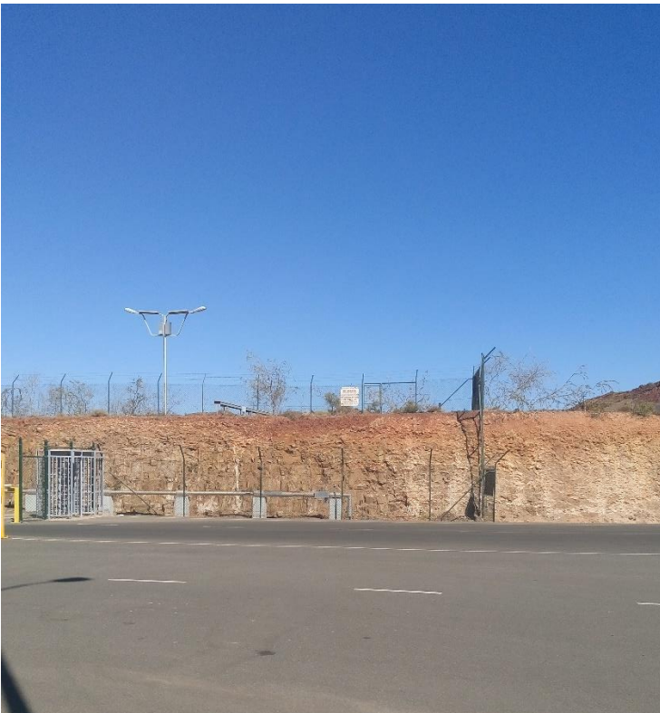
Condition 8: 2.5 m chain link perimeter fence and signage near entrance
