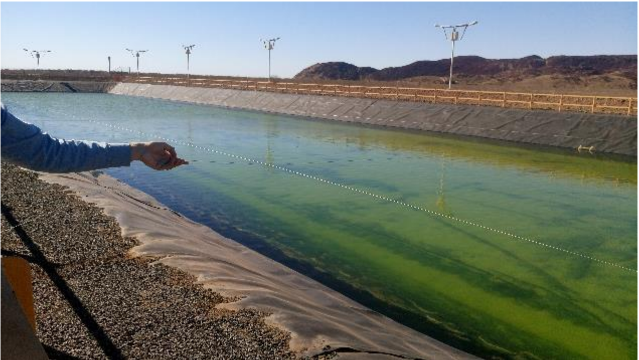
Condition 6: Bird deterrent wires installed over a contaminated water pond
