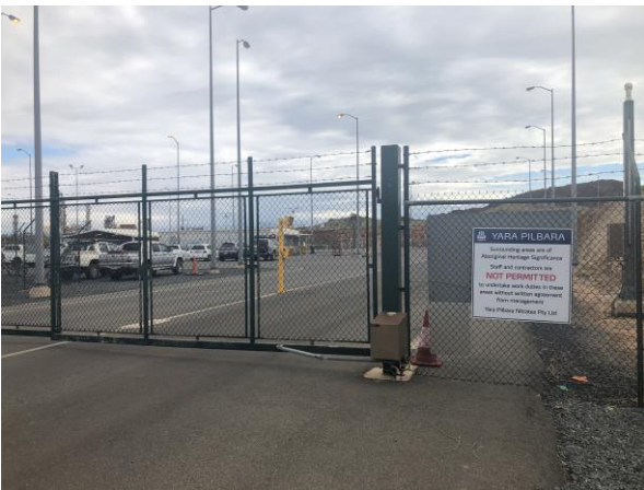
Condition 8: 2.5 m chain link perimeter fence and signage near truck parking entrance/exit
