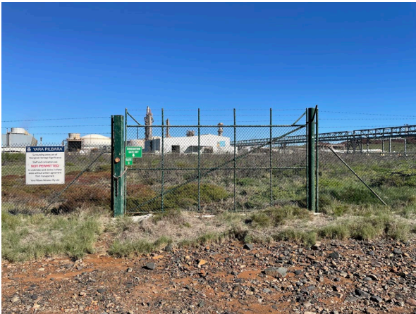
Condition 8: 2.5 m chain link perimeter fence and signage near western perimeter emergency exit (south side)
