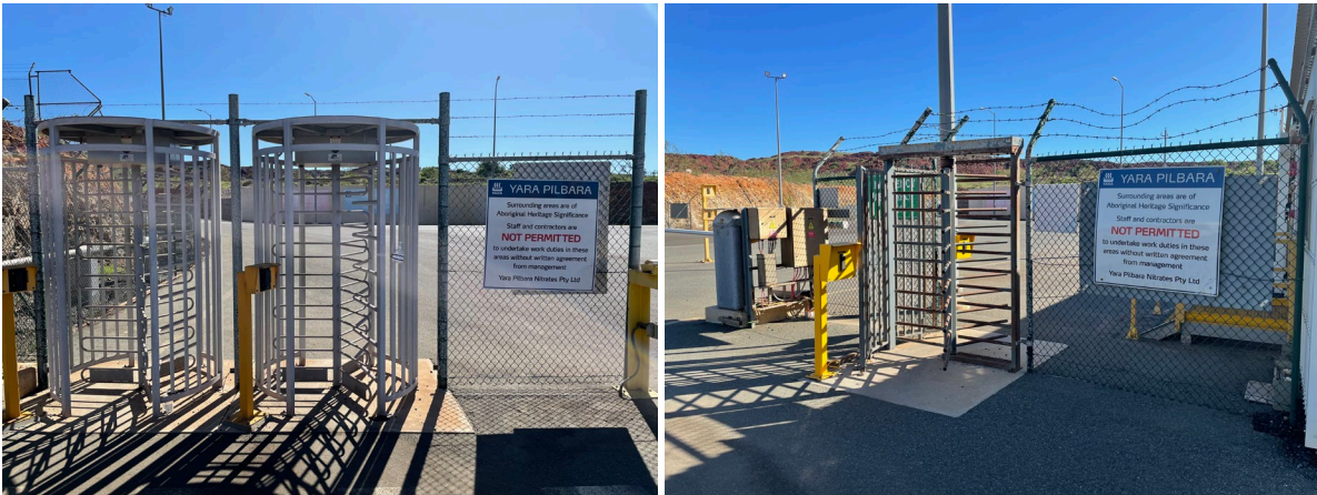
Condition 8: 2.5 m chain link perimeter fence and signage near main entrance/exit
