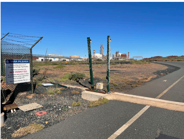
Condition 8: 2.5 m chain link perimeter fence and signage near Integration Road (entrance/exit)
