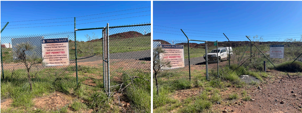
Condition 8: 2.5 m chain link perimeter fence and signage near north western pedestrian gate
