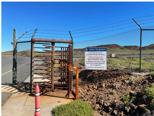
Condition 8: 2.5 m chain link perimeter fence and signage near Integration Road (entrance/exit)
