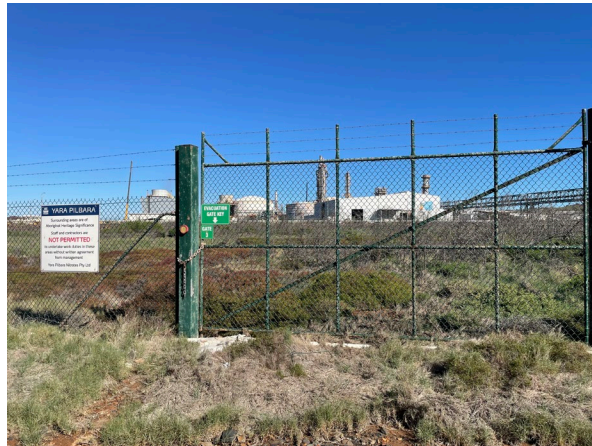
Condition 8: 2.5 m chain link perimeter fence and signage near western perimeter emergency exit (south side)
