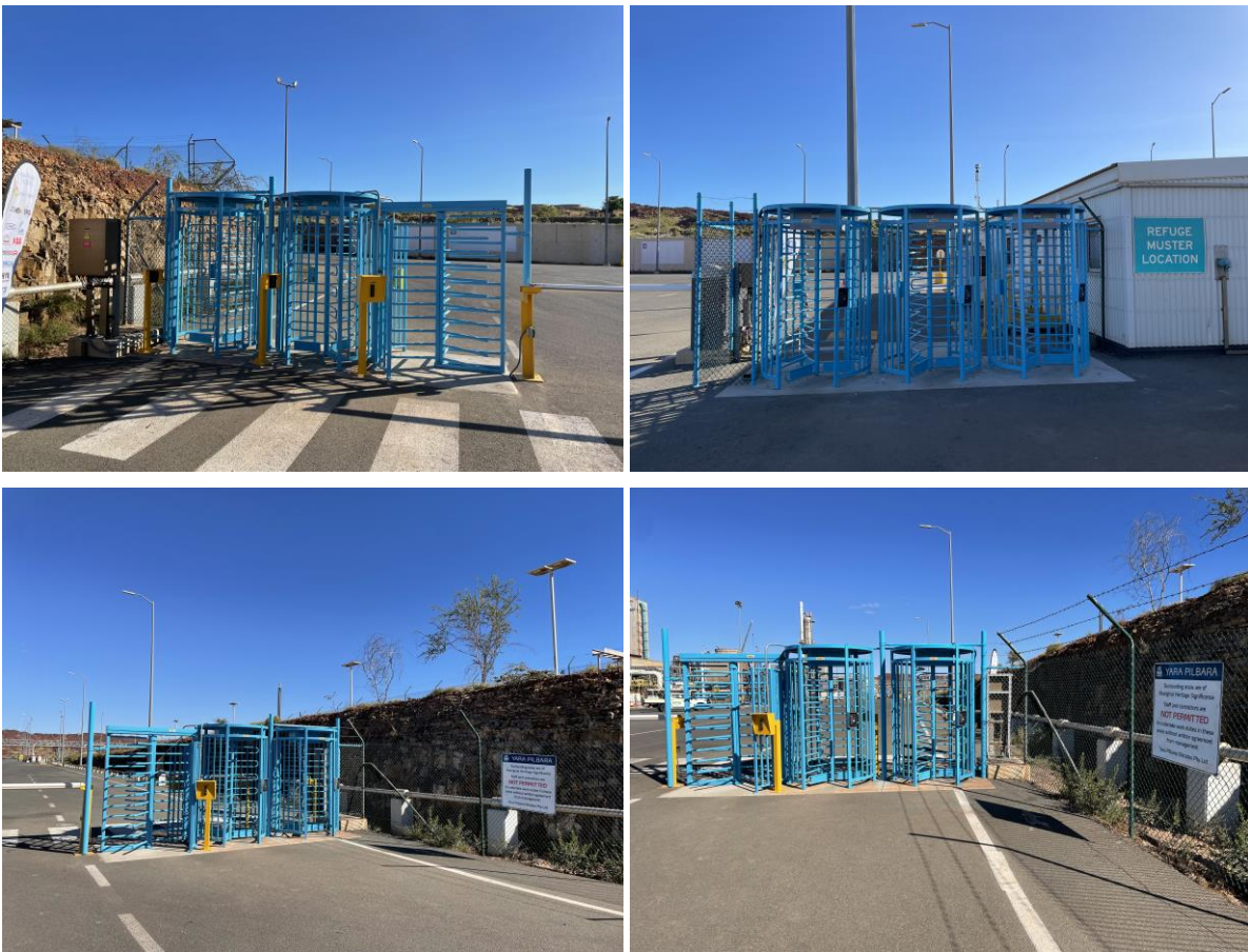
Condition 8: 2.5 m chain link perimeter fence and signage near main entrance/exit-
