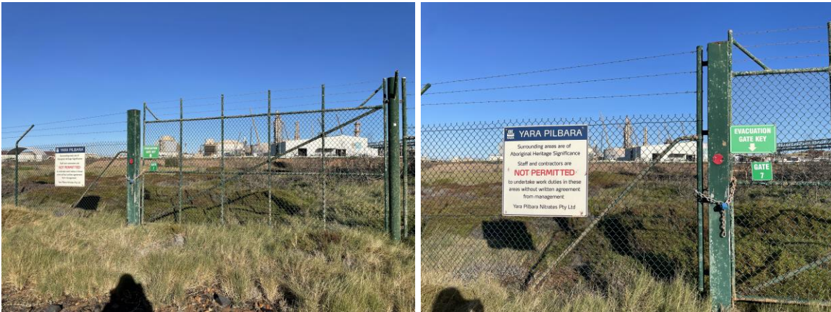
Condition 8: 2.5 m chain link perimeter fence and signage near western perimeter emergency exit (south side)
