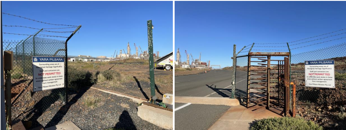
Condition 8: 2.5 m chain link perimeter fence and signage near Integration Road (entrance/exit)
