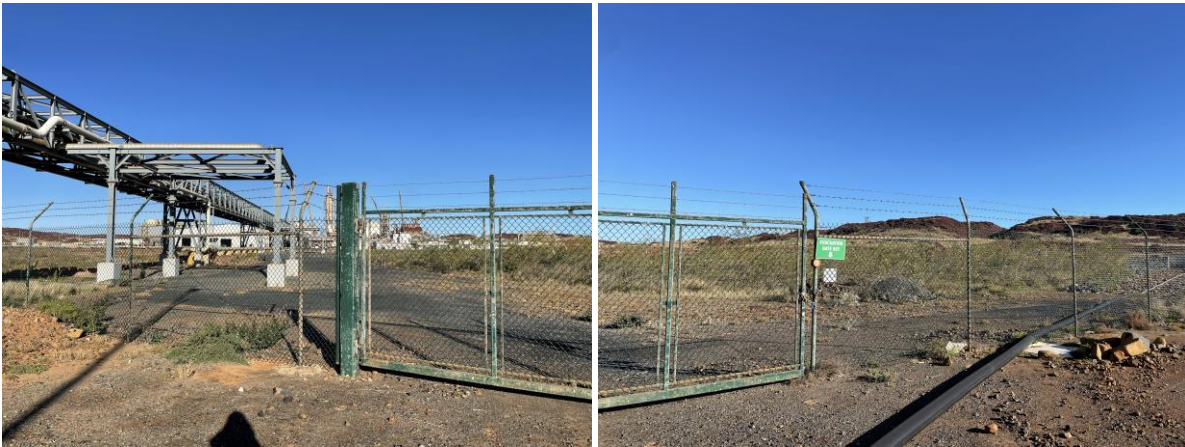
Condition 8: 2.5 m chain link perimeter fence and signage near western perimeter emergency exit (south side)
