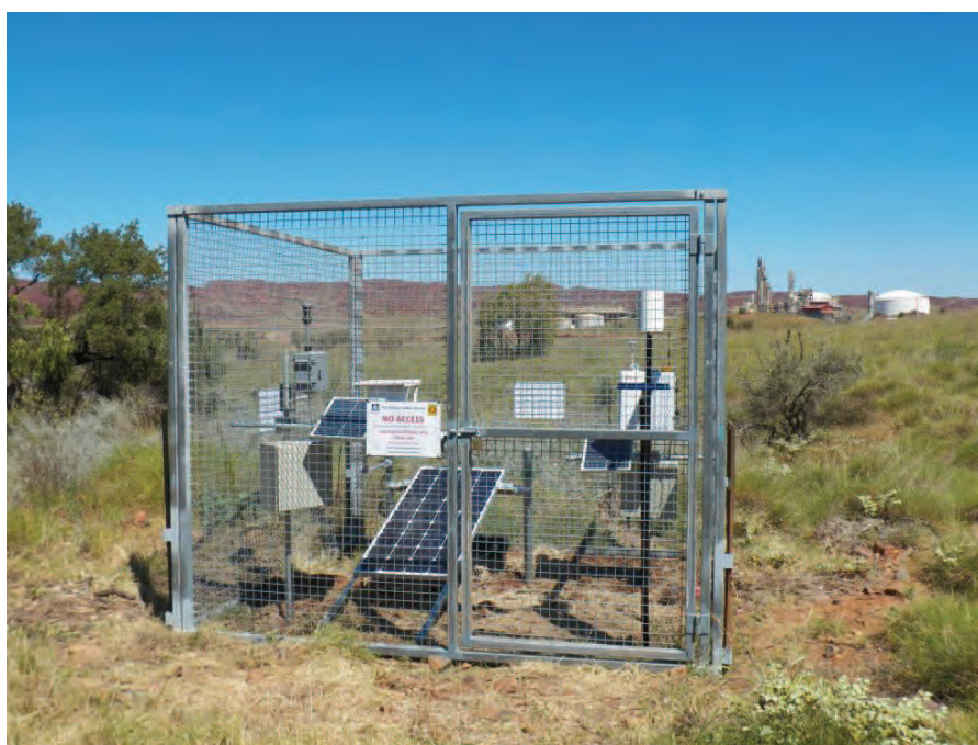
Picture 2.2: Site 6-Water tanks.
