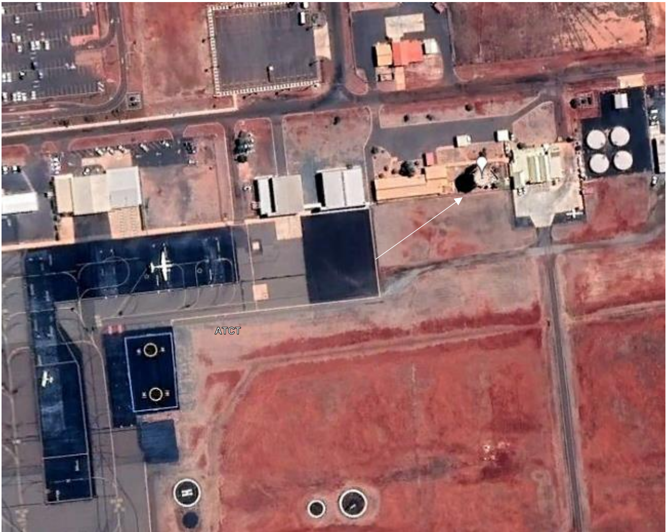
Figure 8 Air Traffic Control Tower observation point receptor
