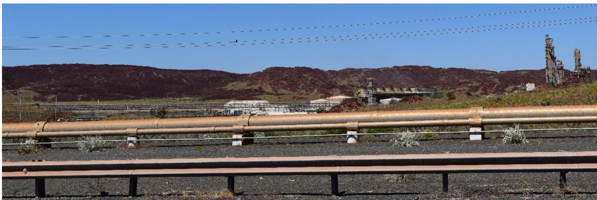
Figure 4-10 VP06 – View south from Village road towards existing fertiliser plant and Project site
