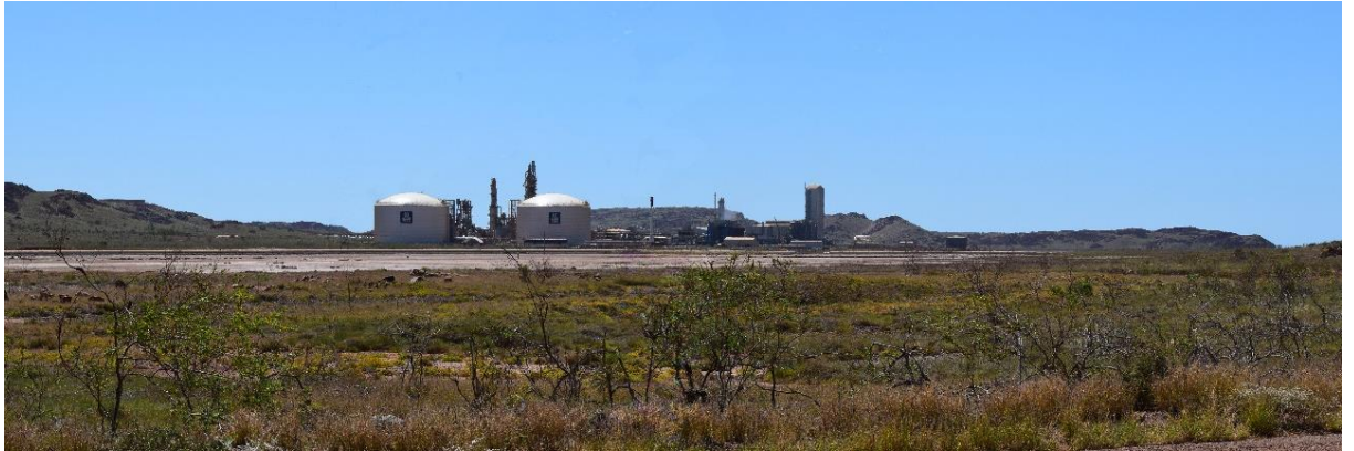
Figure 4-3 VP01 – View north east towards existing fertiliser plant and Project
