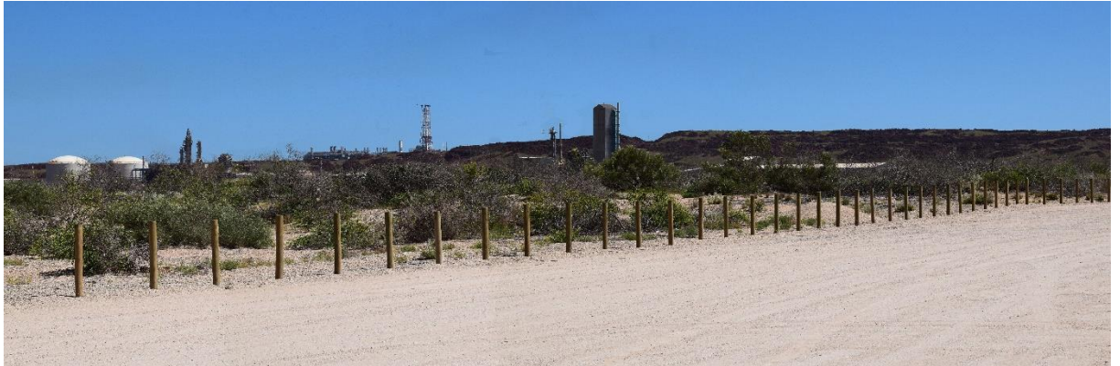
Figure 4-8 VP04 – View west from Hearson Cove towards the Project and existing fertiliser plant
