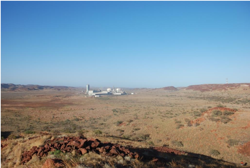
Figure 1: View of the TAN plant from site 22
