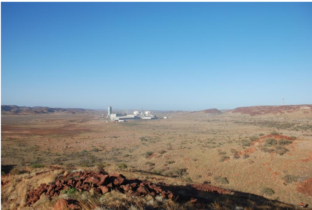
Figure 1: View of the TAN plant from site
